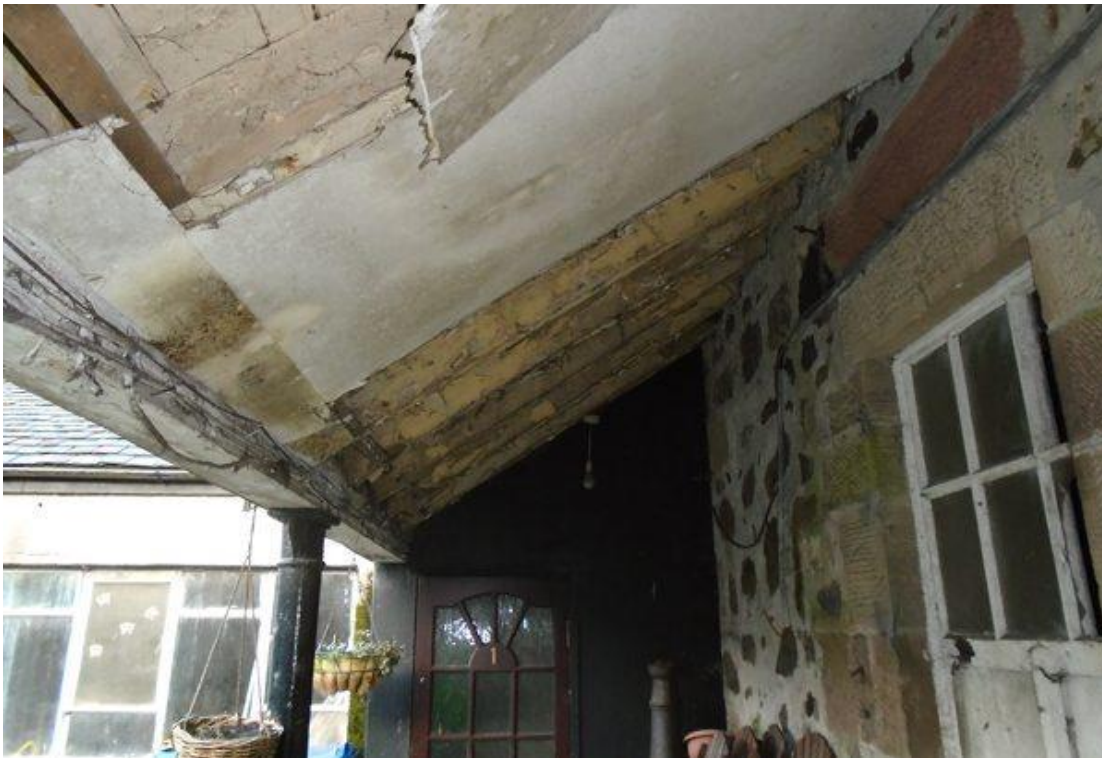
Fig.5 Roof covering walk way. Perimeter beam and rafters have been severely effected by wet rot. Timber lath rendered sloping celing require to be removed.
