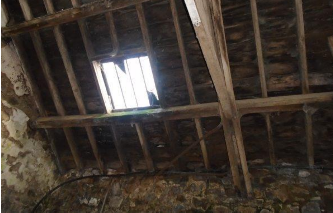
Fig.7 Roof showing main truss and purlins
