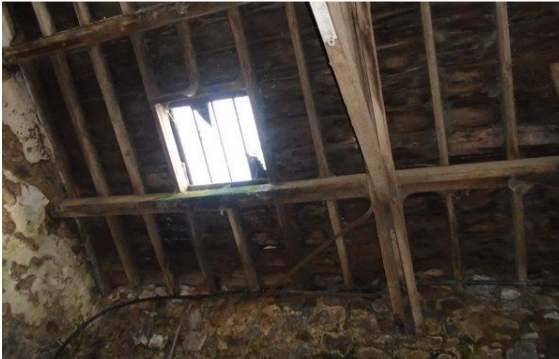
Fig.7 Roof showing main truss and purlins
