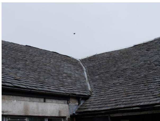
Figure 3 – Lifted Flashing on Roof of Building.
