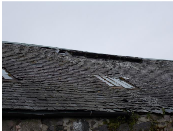
Figure 5 – Raised and Missing Tiles on Building.
